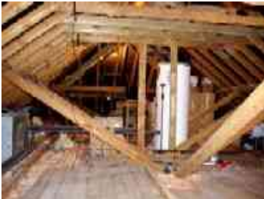
Antenna and Attic installation
